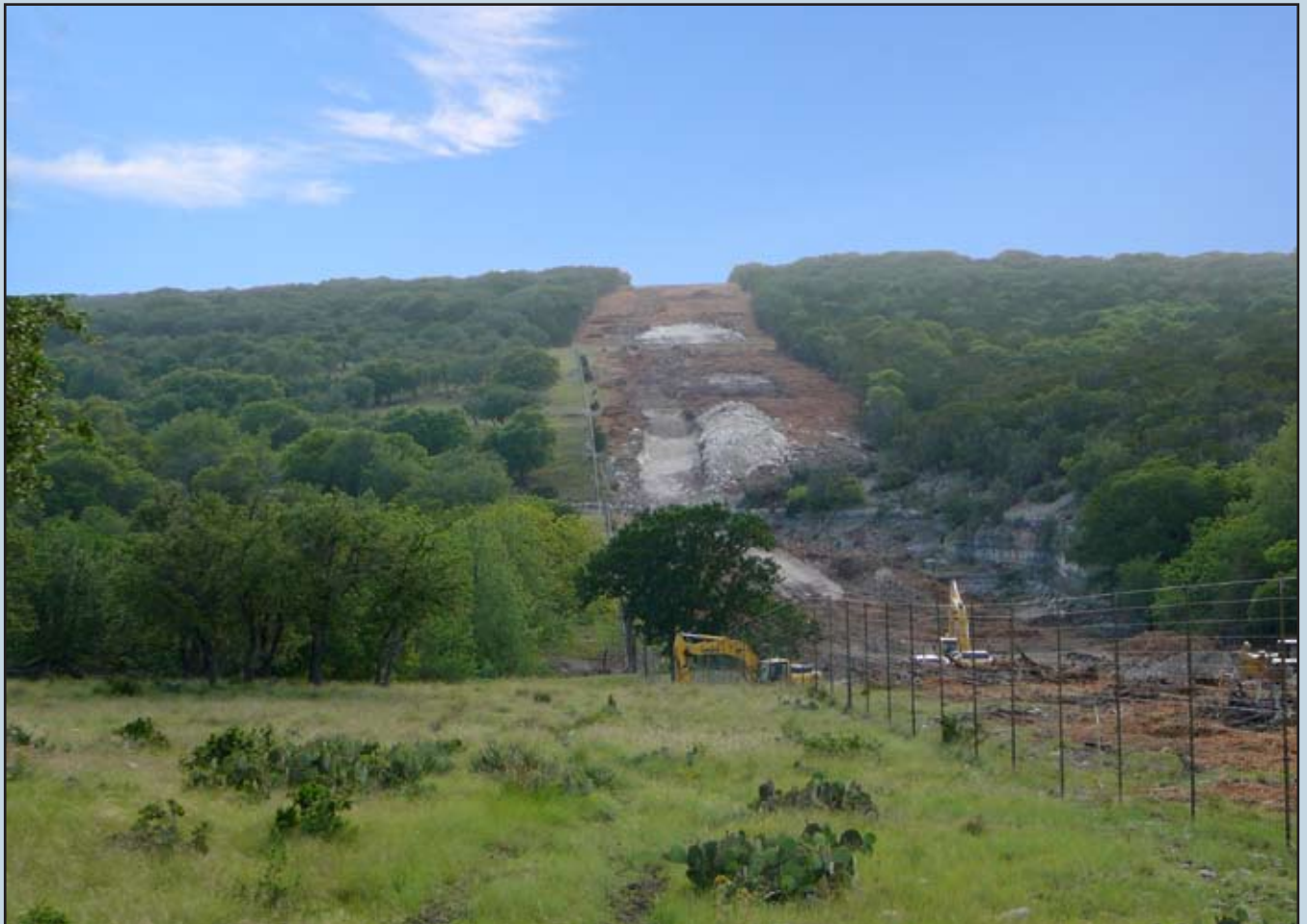
actual construction of FPL private wind energy line near Harper, TX 2009
