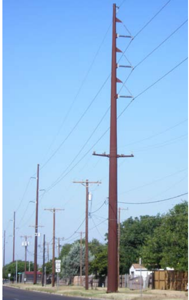
corten steel monopole perma-rust surface
