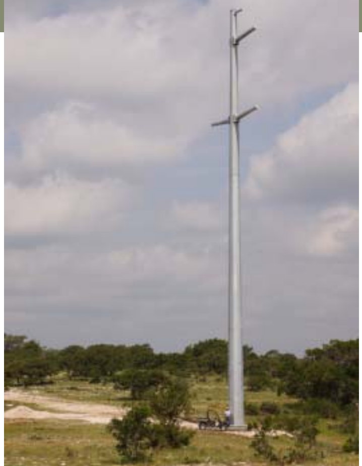
Towers have to be big to support 345kV lines. Some are made of concrete, others are made of galvanized metal. The six-foot, 200-pound man and ATV next to the tower in the right photo give a sense of scale.
